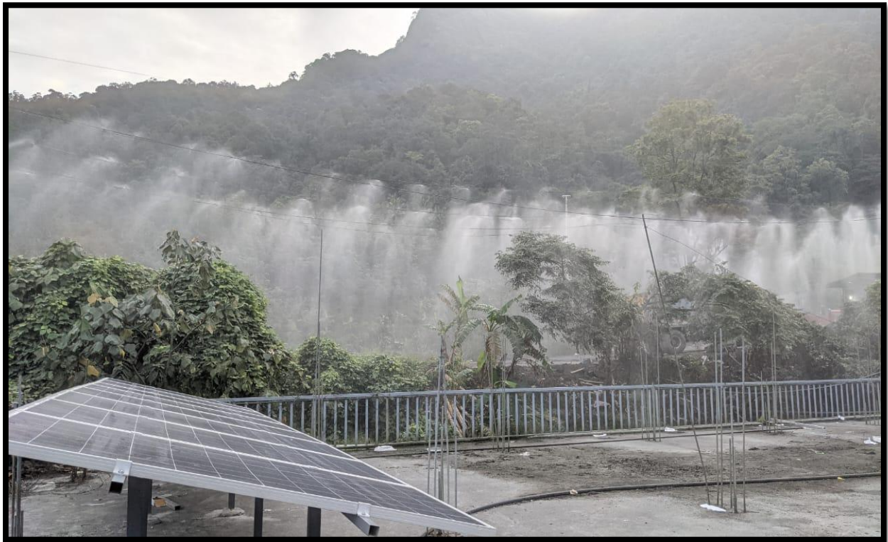
Sprinklers in the Quarry Site
